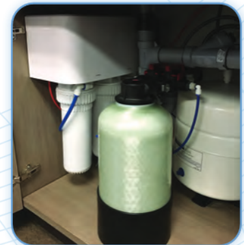
25020189 Kit, Tank, Recirculation, H.E.R.O.™ Applied when the H.E.R.O.™ is installed under a kitchen sink or in a slab home without a basement. This tank provides blending of the HERO recirculated water and helps keep the system operating at its peak performance.
